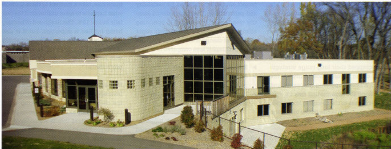
LAST YEAR, CONSTRUCTION RESULTS CORP. FINISHED AN ADDITION AND RENOVATION TO ST. BARNABAS CHURCH IN PLYMOUTH, MINNESOTA. CONSTRUCTION RESULTS RECENTLY ABSORBED THE CLIENTS, RECORDS, AND EMPLOYEES OF ONE OF ITS CHIEF RIVALS, OLSON GENERAL CONTRACTORS.
