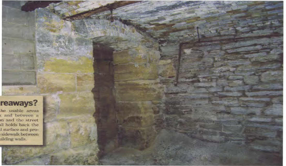
Under the ground at 250 Third Ave. N. in Minneapolis, an areaway was cleared and refilled to improve aboveground access to the Minnesota Twins' new stadium, Target Field. (Submitted photo: Paul Ormseth)
